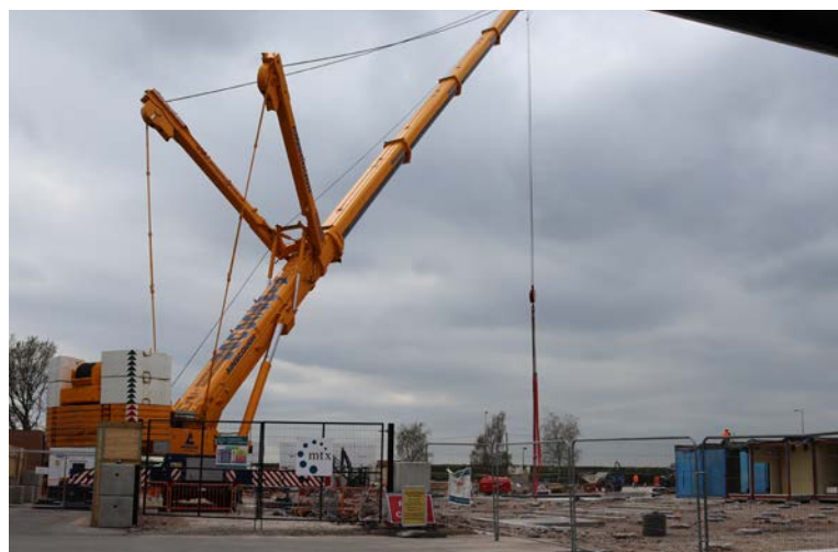
Work starts on Leighton Hospital's new Accident and Emergency Department, just one of the Trust's investments in its infrastructure
